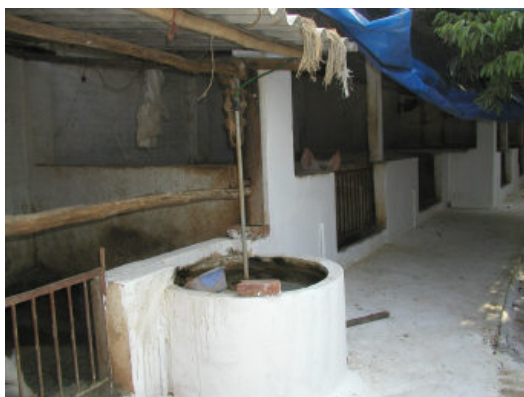
Biogas production on a small pig producing farm in Bac Giang
